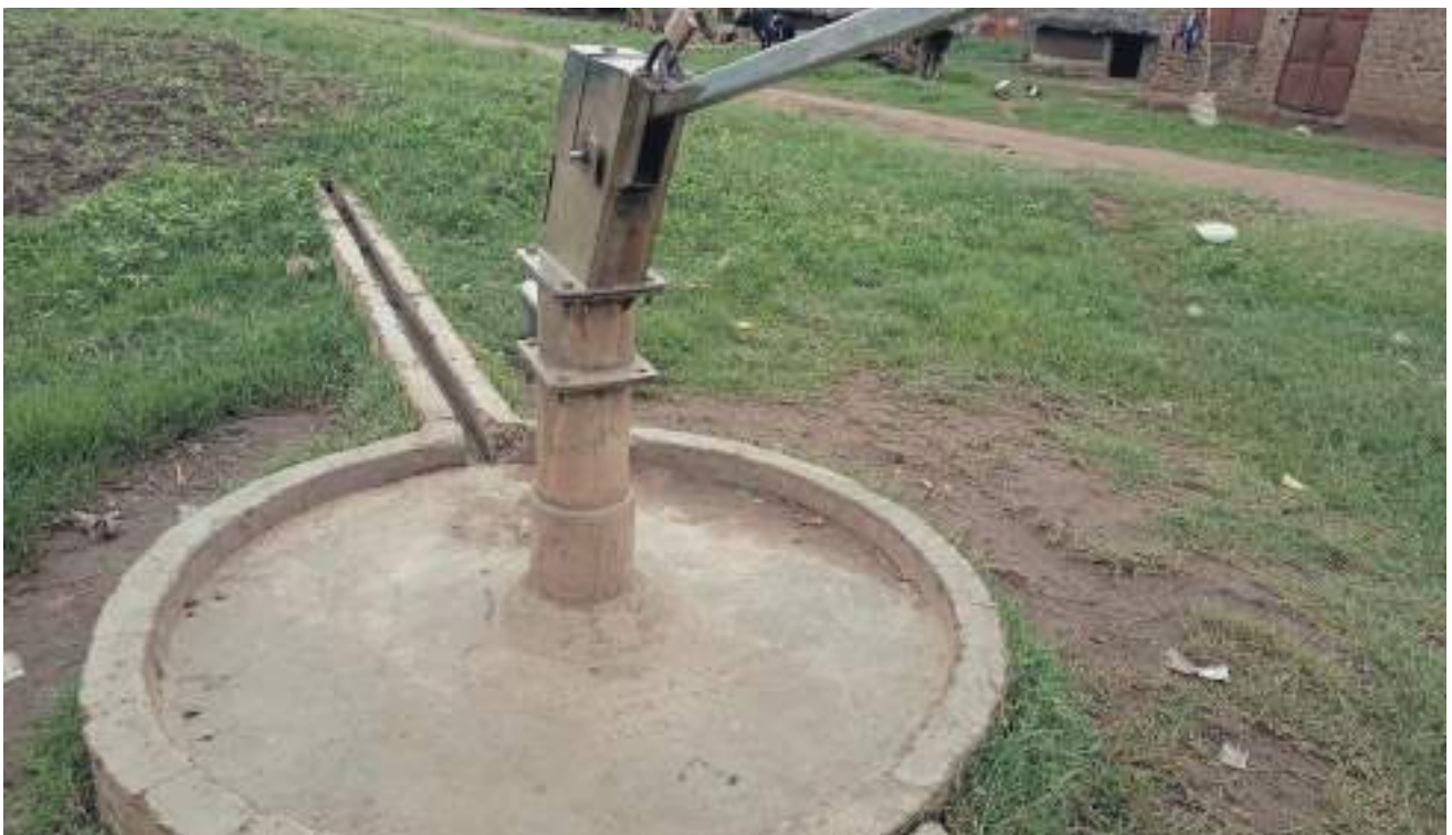
Anon functional borehole in one of the town councils of Agago
